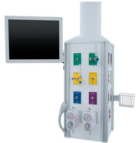
Figure 5: Gas outlets on a mobile boom attached to the ceiling.
