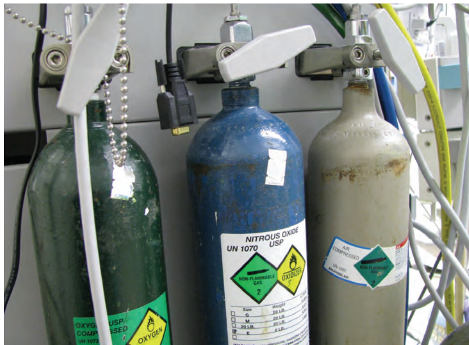
Figure 1: From left to right, properly colored and labeled oxygen cylinder and nitrous oxide cylinder next to a gray, improperly colored medical air cylinder that should be yellow.
